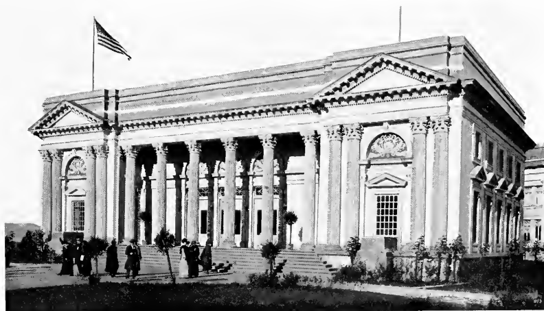
THE UTAH BUILDING
